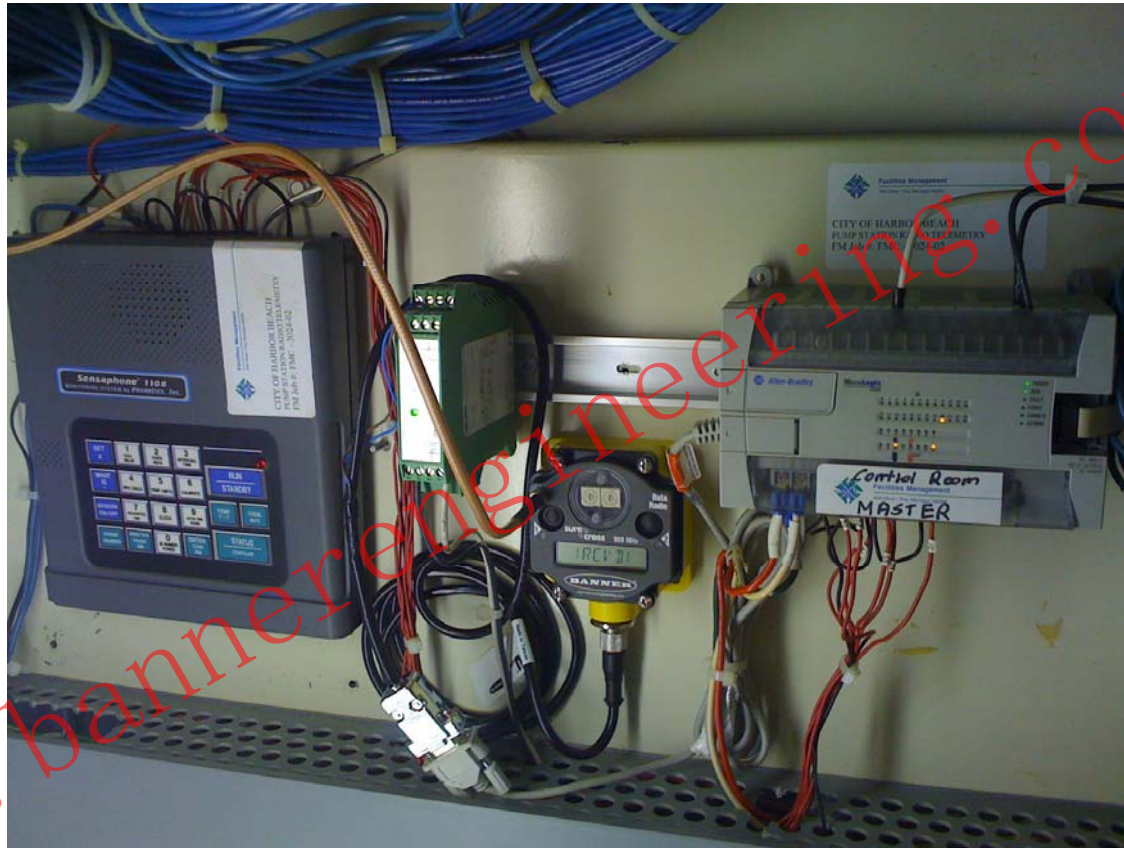
Micrologix PLC Integration via AB DF-1
